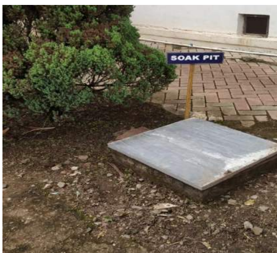
Figure 4: Soak pit for chemistry lab discharge
