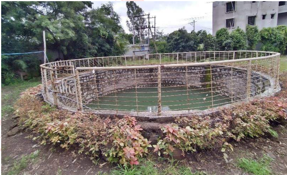
Well protected open well
